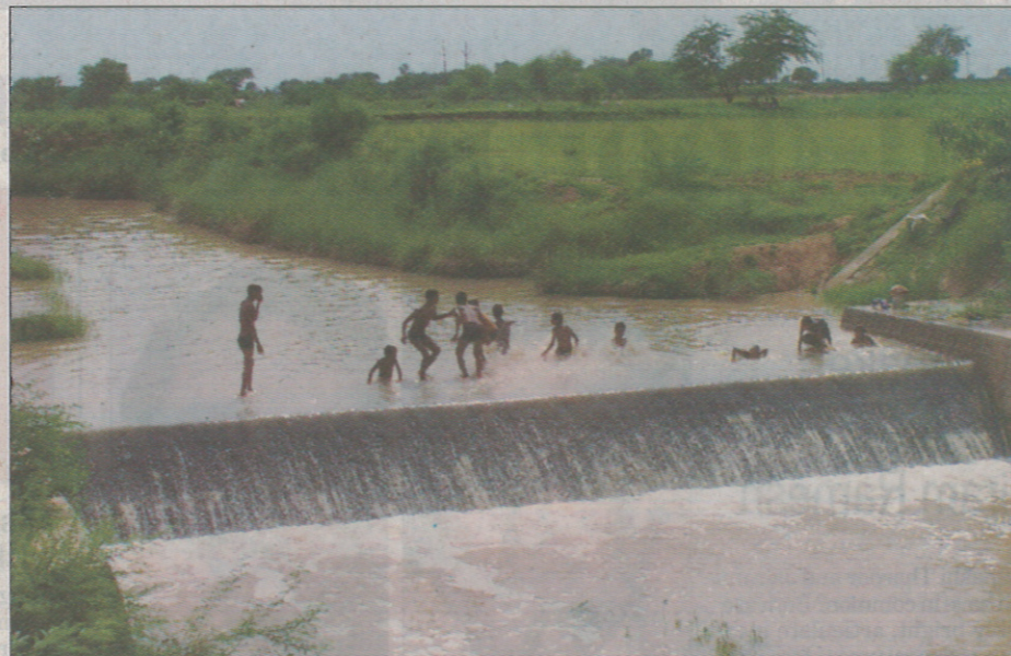
■ JOY OF WATER-HARVESTING: Here is a new checkdam built in Ganeshgarh village in Jhansi, which is a miniature of Chandela-Bundela period dams.
